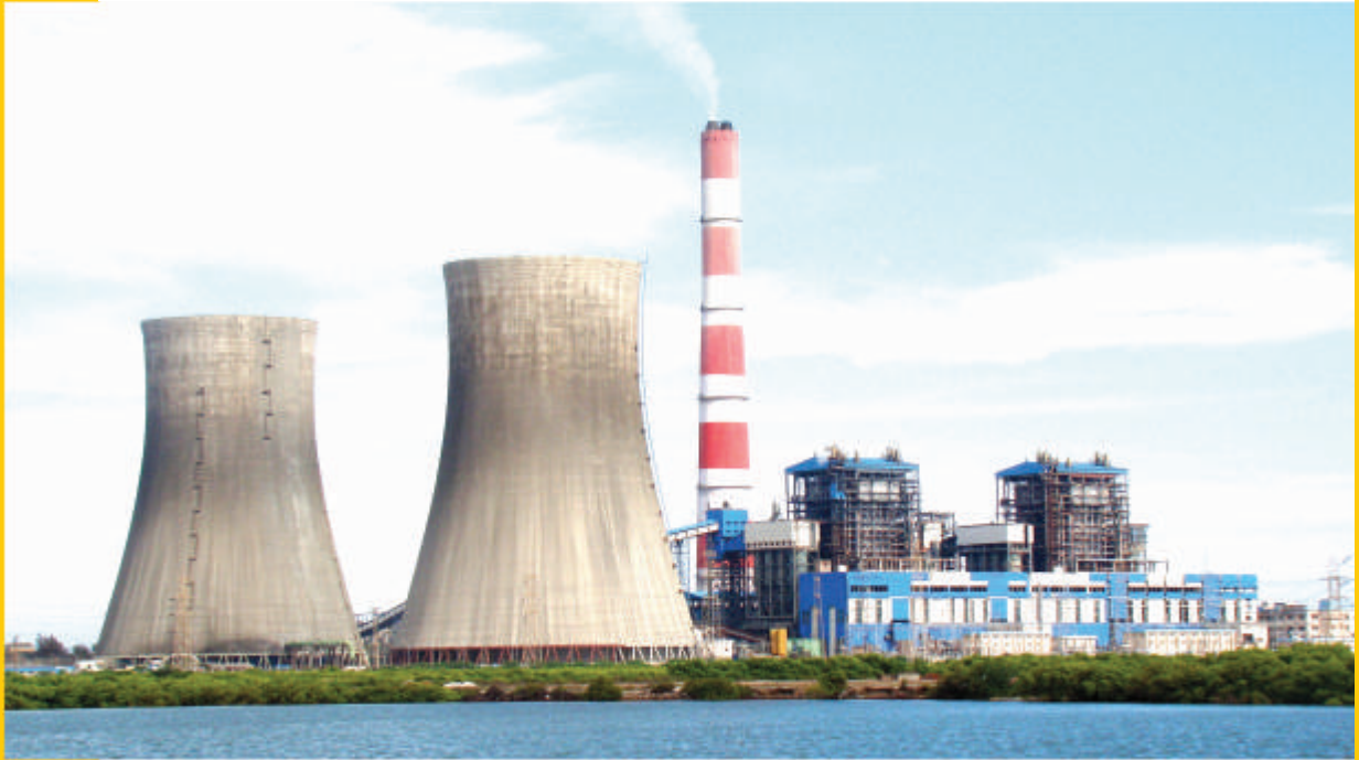
Panoramic View of the Plant
