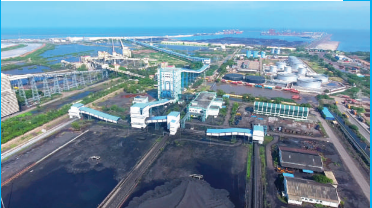
Coal Stock Yard
